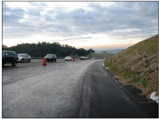
Eastbound US 50 HOV Lane Construction near Bass Lake Road
