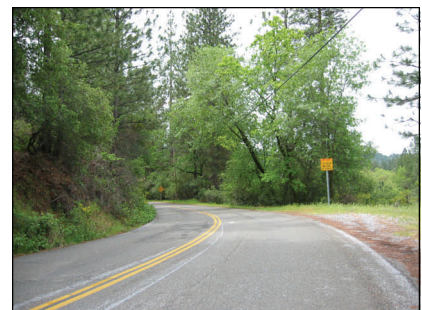
Carson Road Before 2010 Rehabilitation
