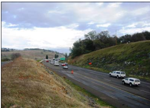
US 50 HOV Lane Under Construction
