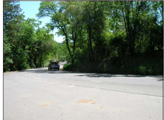
Cold Springs Road after ARRA road rehabilitation
