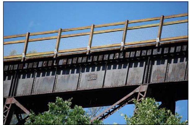
El Dorado Trail Weber Creek Trestle Bridge
