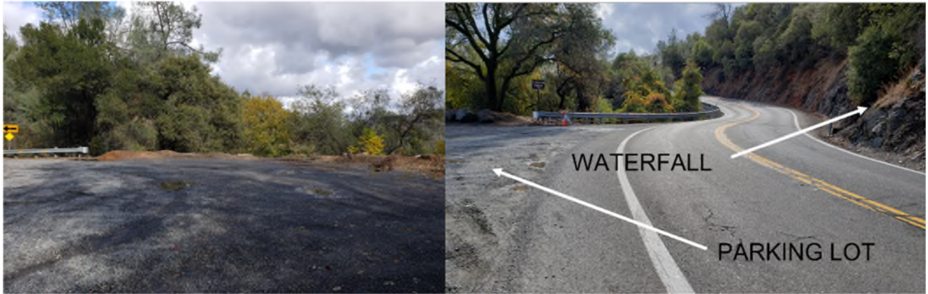
FIGURE 43: PHOTO OF SR 49 AT CANYON CREEK EASTBOUND
