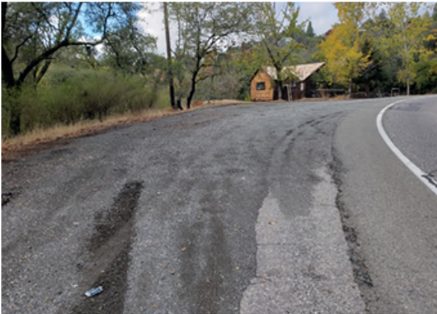
FIGURE 38: PHOTO OF SR 49 NEAR PM 2.0 EASTBOUND
