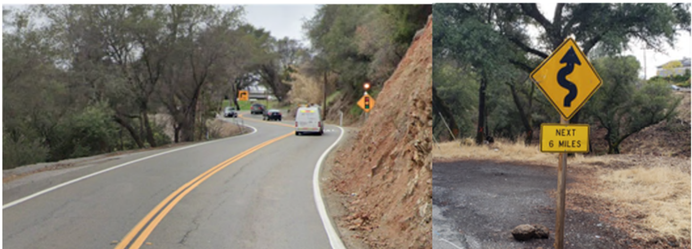
FIGURE 36: PHOTO OF SR 49 NEAR LINCOLN WAY SIGNAL (LEFT - WESTBOUND, RIGHT - EASTBOUND)
