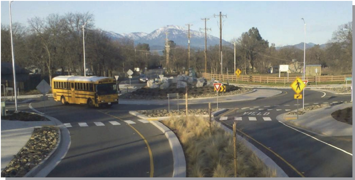
Roundabout Intersection Control
