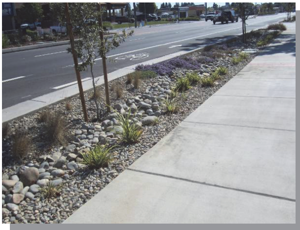
Streetscape planting incorporating storm water swale
