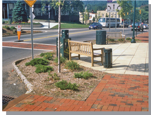
Decorative street crossings with bulbouts make it easier for drivers to see pedestrians and shorten the crossing distance.
