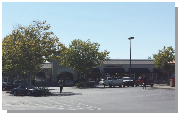
There are no clear pedestrian routes from parking to stores
