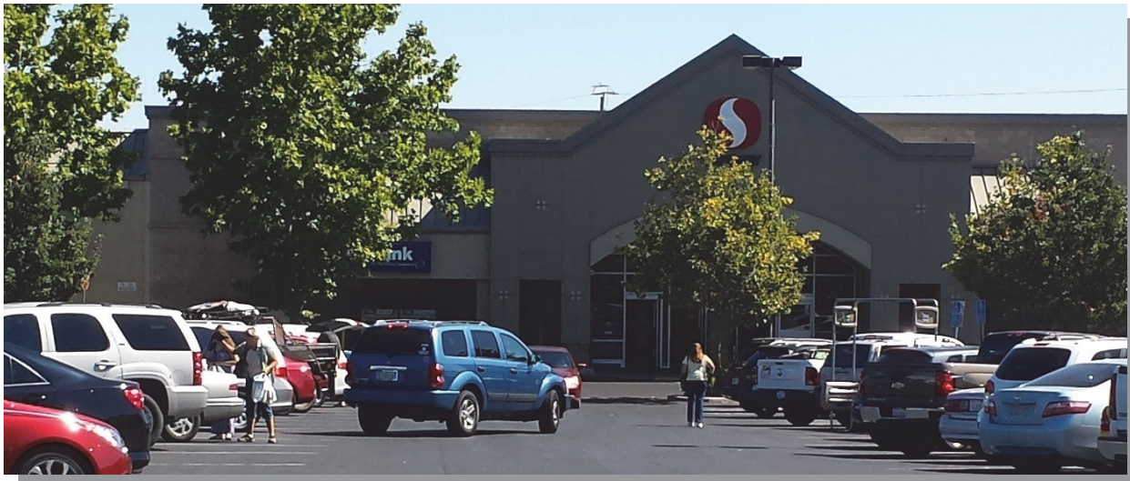
Potential for safety issues when drivers and pedestrians must compete for travel space.
