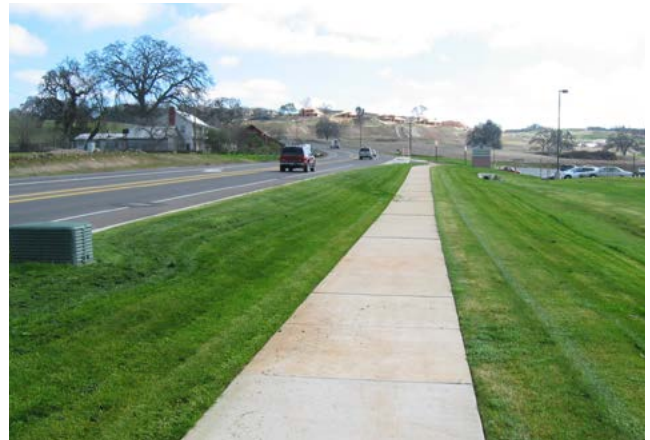
A separated sidewalk along Green Valley Road in front of Pleasant Valley School provides a safe and comfortable walking experience for users.
