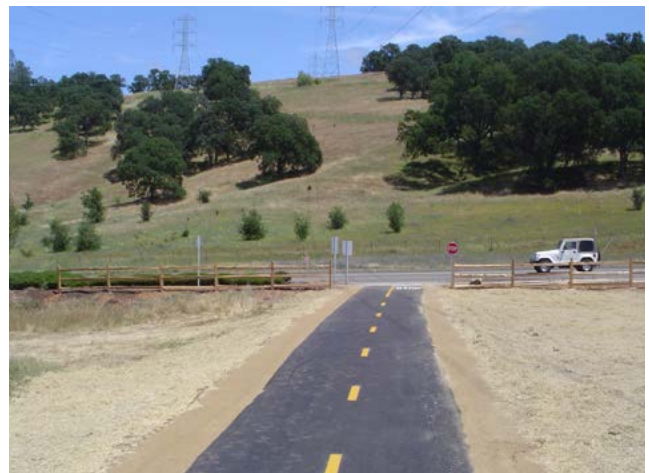
The New York Creek Trail, a Class I Shared Use Path in El Dorado County
