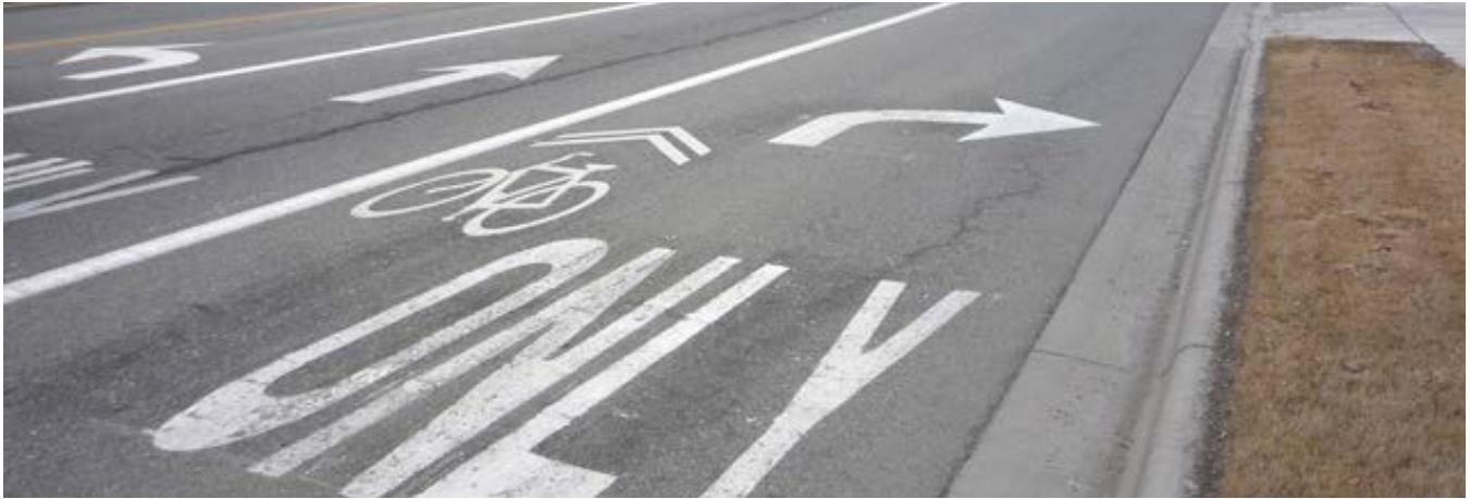
Shared lane markings and signs indicate that bicyclists should right in the left side of this right turn only lane.
