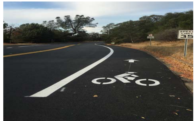
Example of a Class II Bicycle Lane on Ray Lawyer Drive
