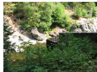
The missing Brockliss Bridge
