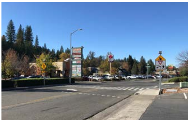
Figure 6-10: Example of an RRFB in Placerville
