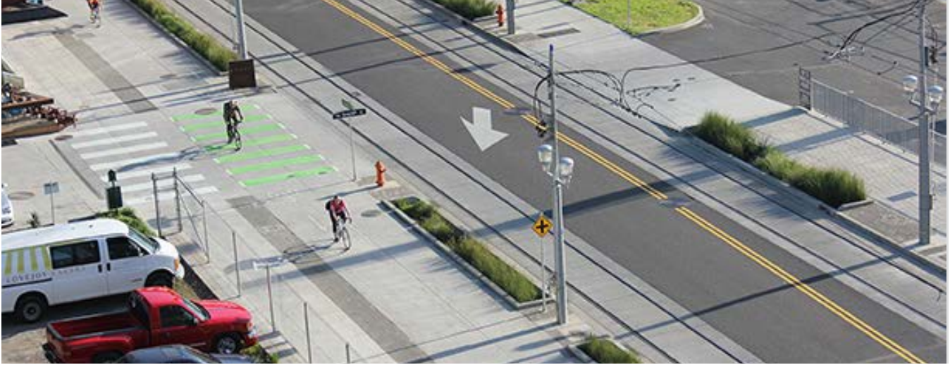
Intersection crossing markings can be used at signalized intersections or high volume minor street and driveway crossings.
