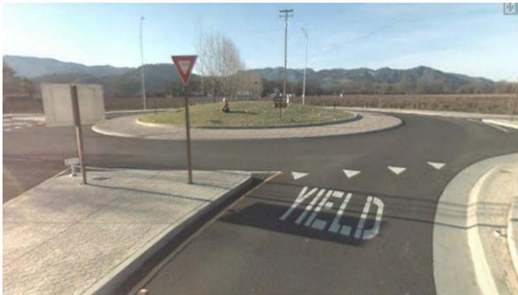
Ground View 36 District 1, Mendocino County, Hopland, CA - SR 175 and Main Street
