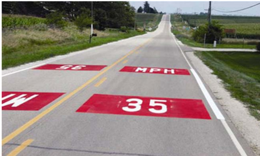
Figure 12. Enhanced speed limit markings (FHWA-HRT-08-067)
