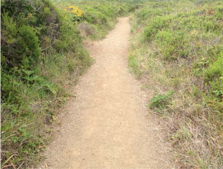
Figure 22. Path with crushed granite surface.
