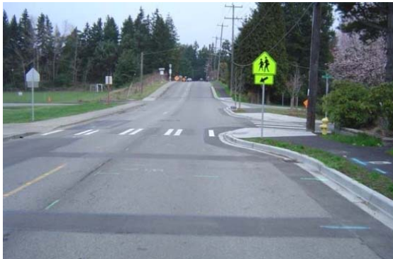
Figure 4. Curb bulb-out
