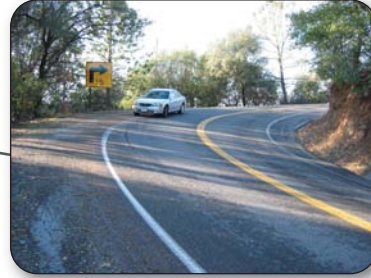
Tight Curve on Existing SR 49 Alignment
